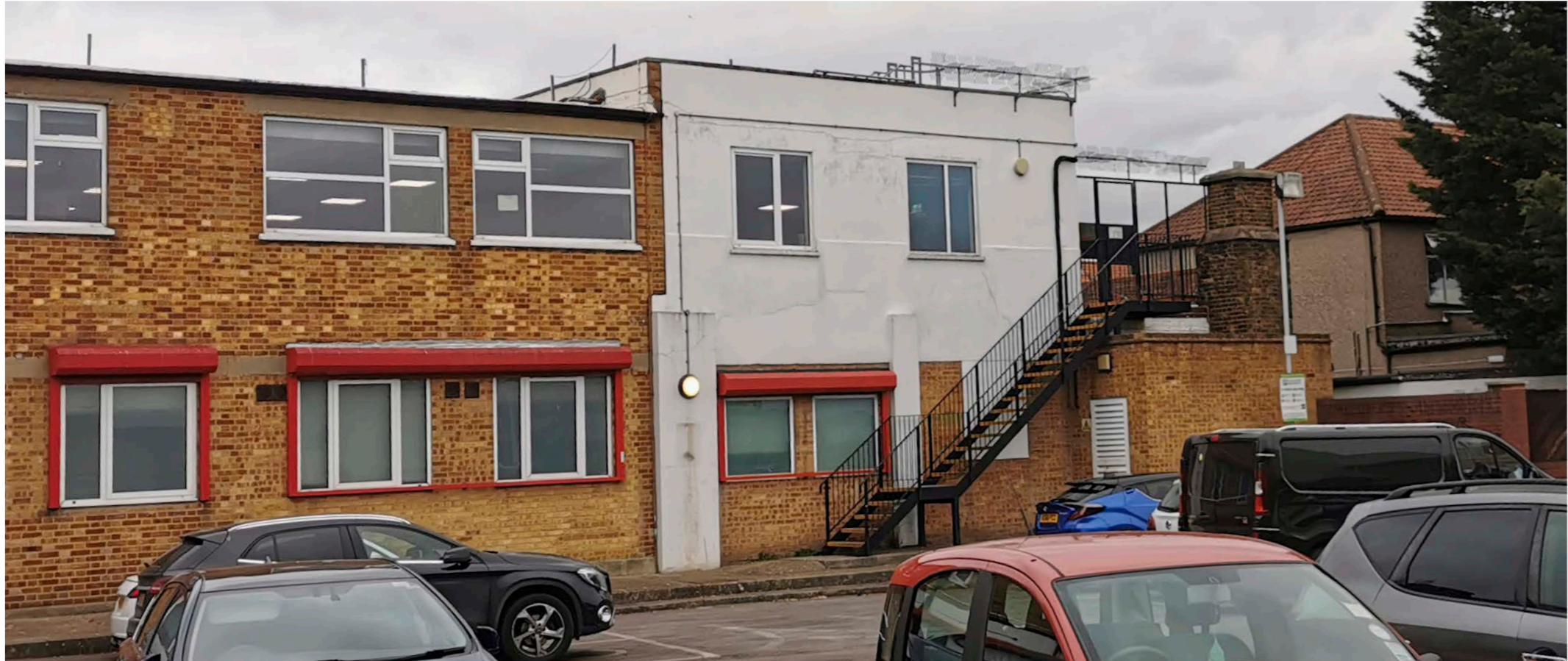
Part south elevation - escape stair & boiler rm. detail, shutters raised
