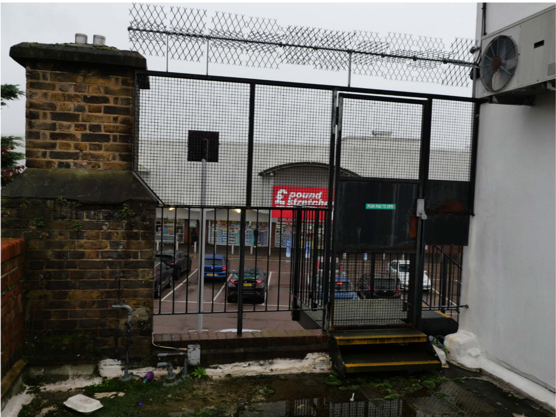
1st fl. roof terrace to east showing security screen on fire escape route with plant room chimney
