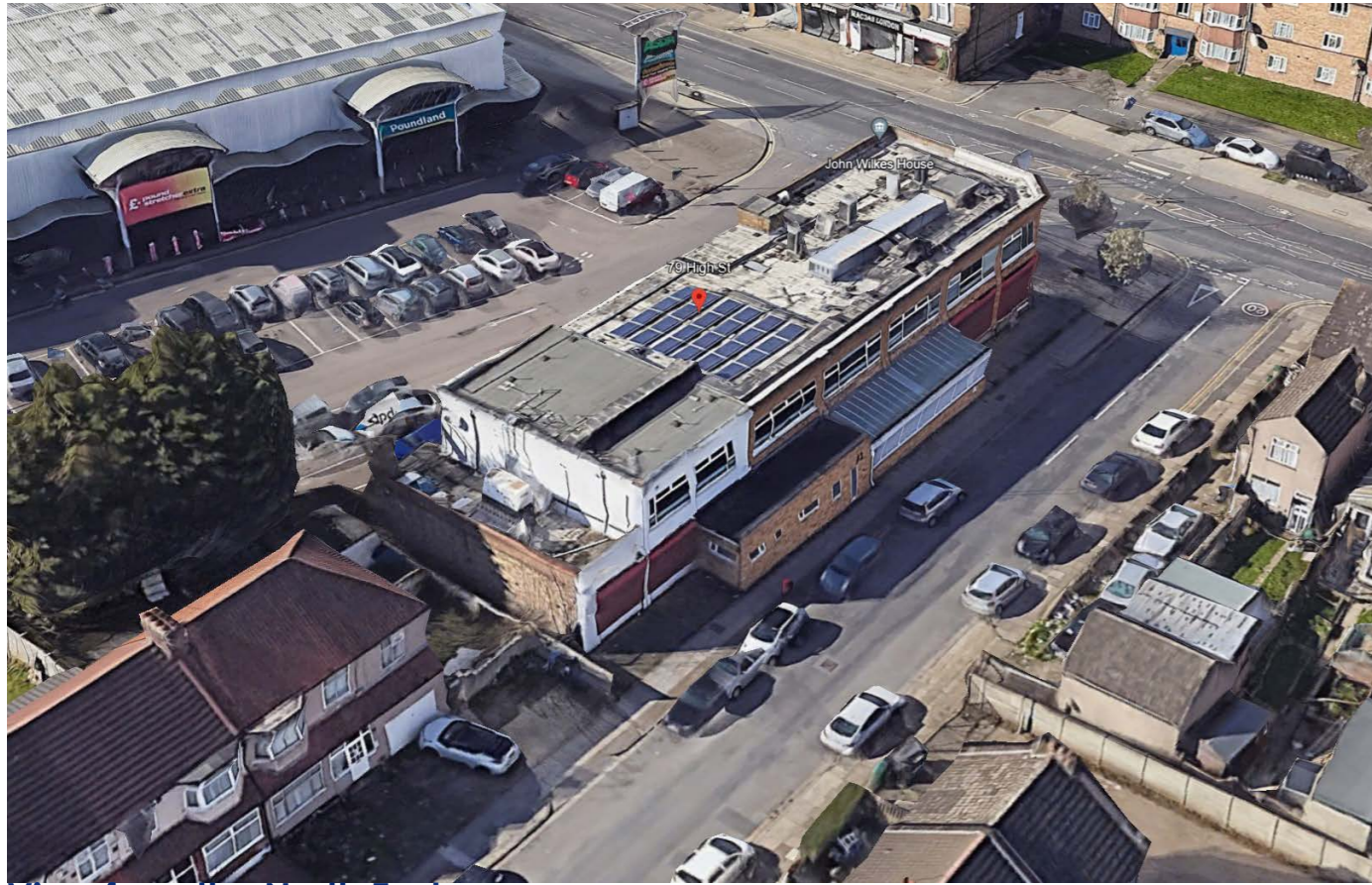
View from the North East
