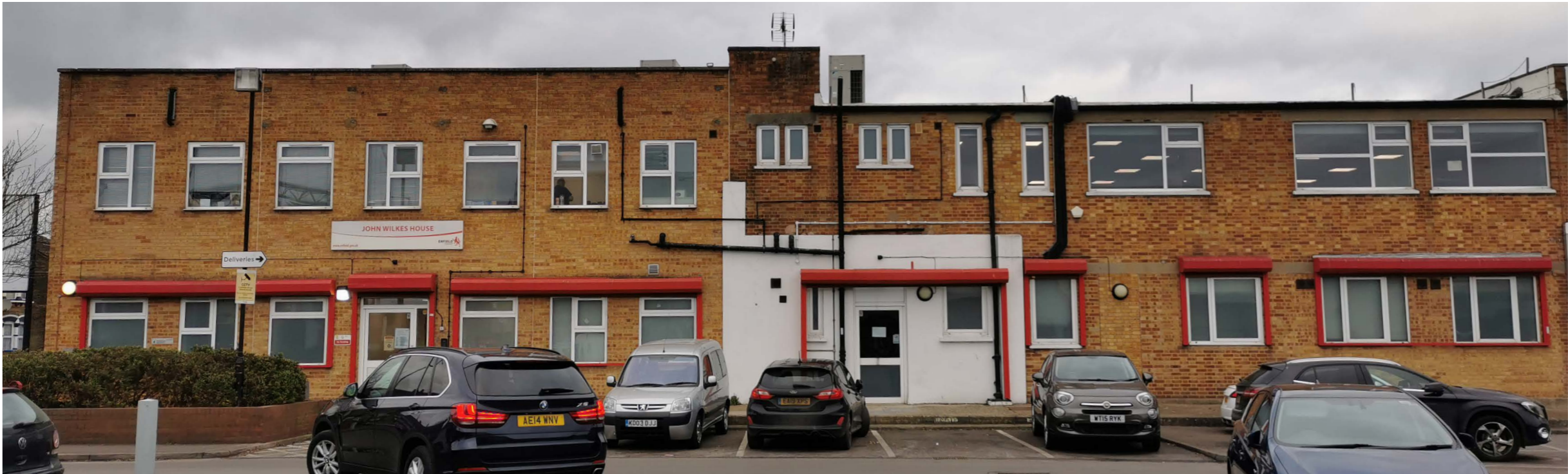
Part south elevation - shutters raised
