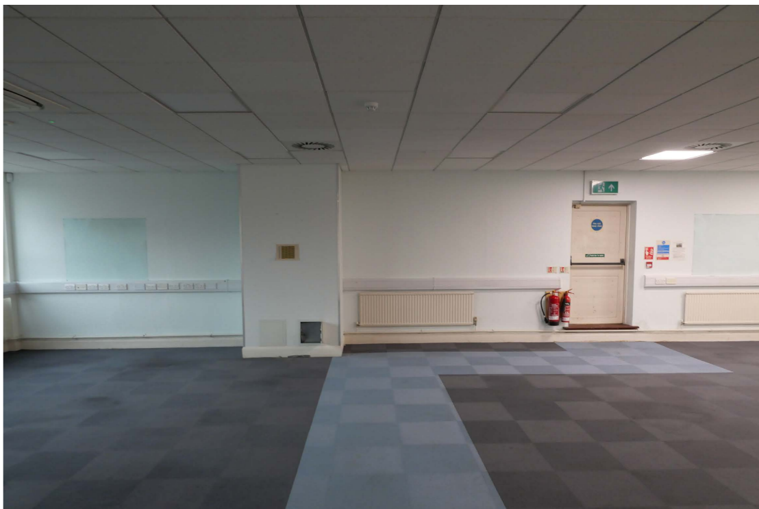
1st. fl. interior east gable with existing fire escape
